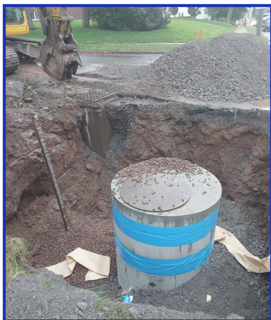
Image of a sanitary manhole.
